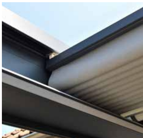
Waterproof folding roof that can be retracted to any position
