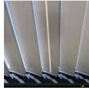
Ledstrips in louvers
